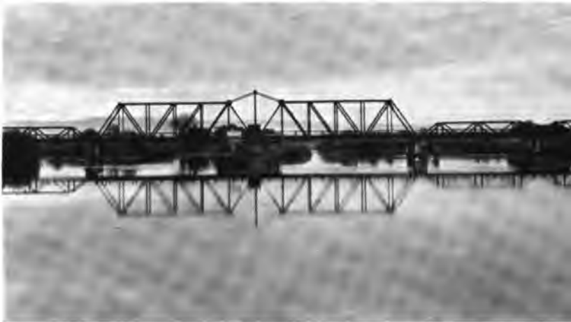
Middle River bridge on Borden Highway west of Stockton.
